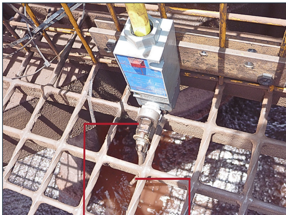
Extended Arm to Rake Tag (through Grid Mesh)
